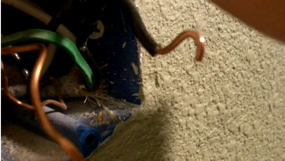
Properly Formed Hot Wire
