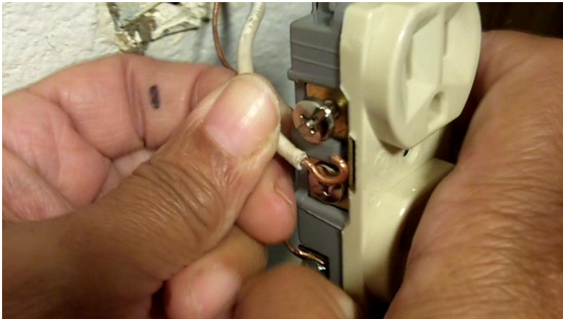
Attaching the neutral wire
