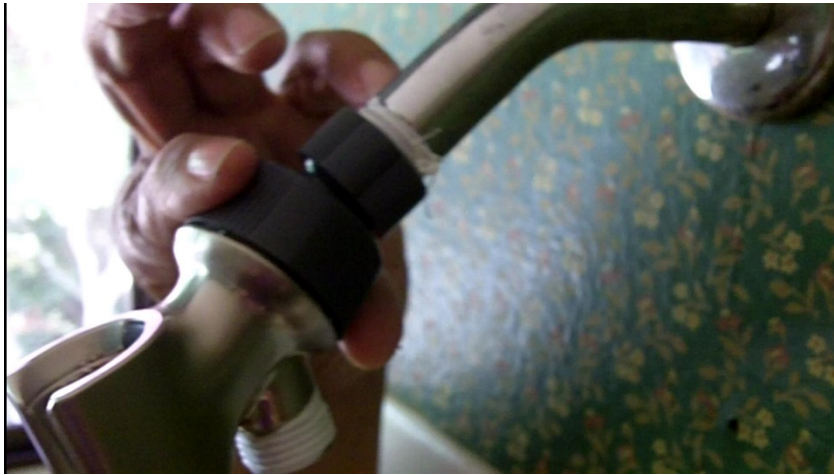
Attaching the showerhead holder
