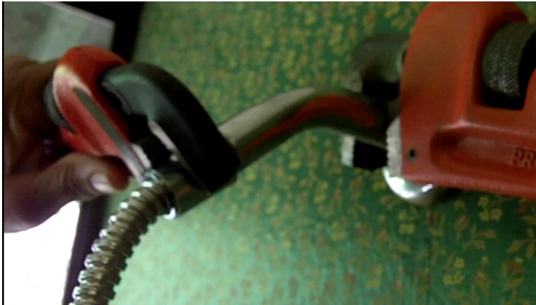
Removing existing showerhead with pipe wrenches
