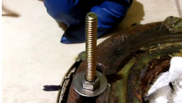
Installed Flange Bolt with Nut and Washer
