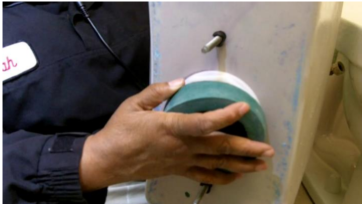
Installing Tank Gasket
