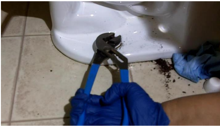
Removal of the Rusted Bolt with Channel Locks
