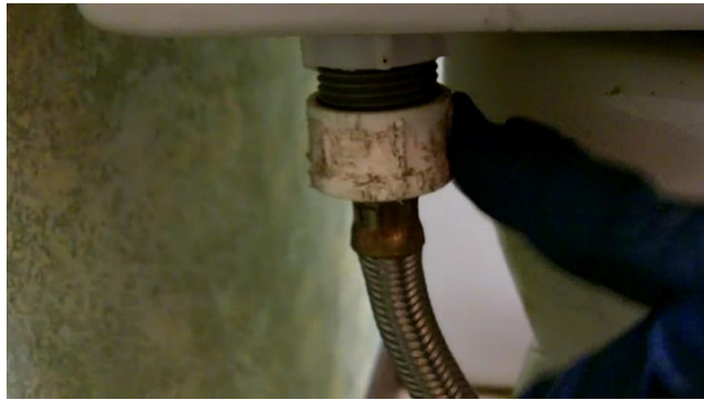
Water Supply Line Connection to the Tank
