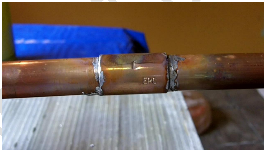
Completed solder job
