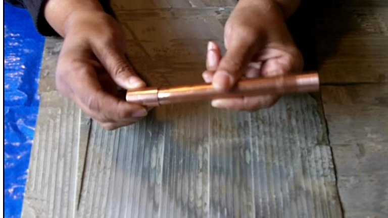
Assembling Copper pipe and fitting
