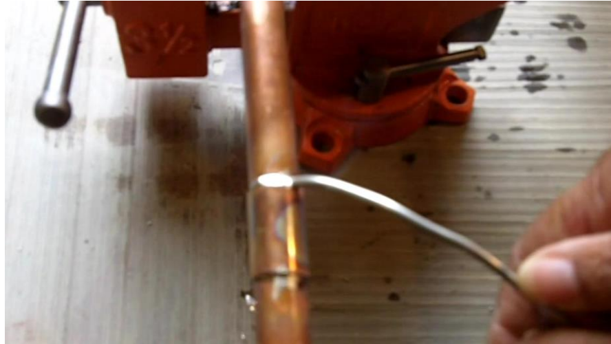
Applying the solder
