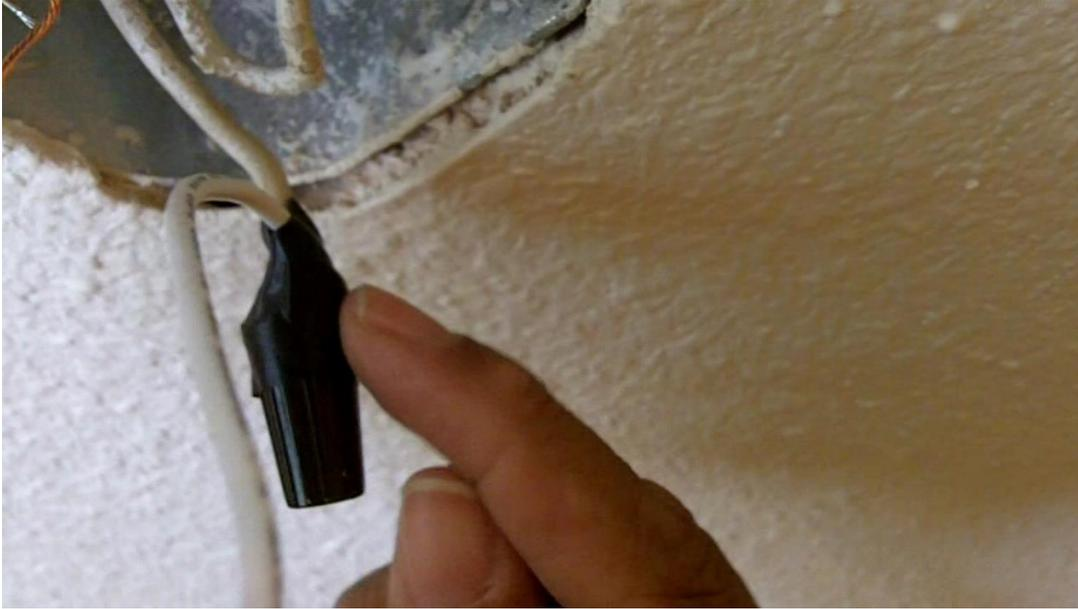
Wires wrapped with electrical tape
