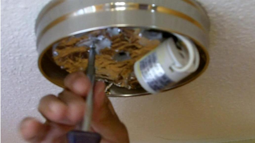
Tightening the screws to secure the fixture
