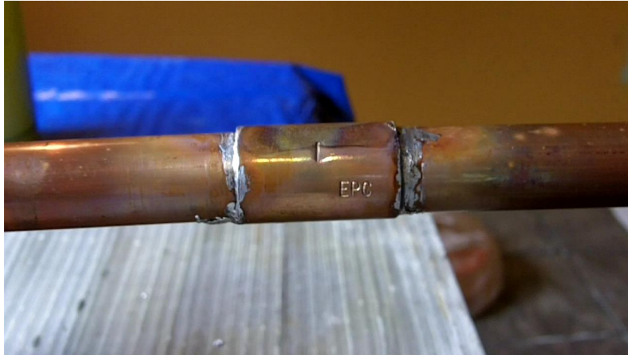
Completed solder job
