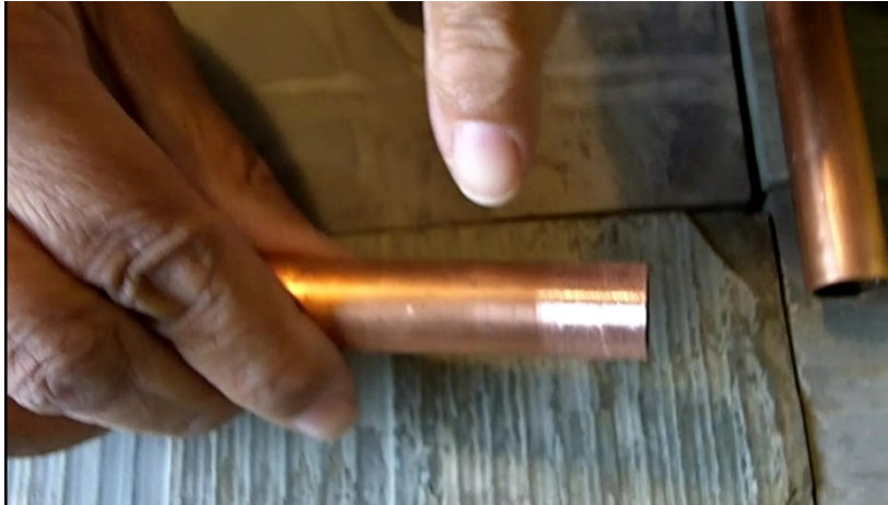
Copper pipe with the end cleaned for soldering
