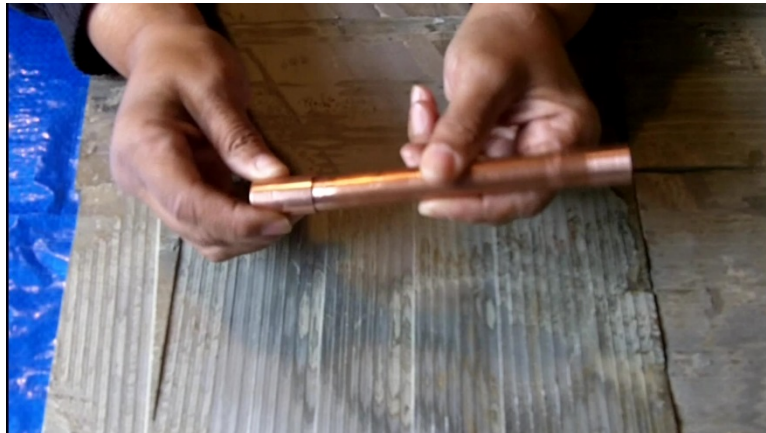
Assembling Copper pipe and fitting
